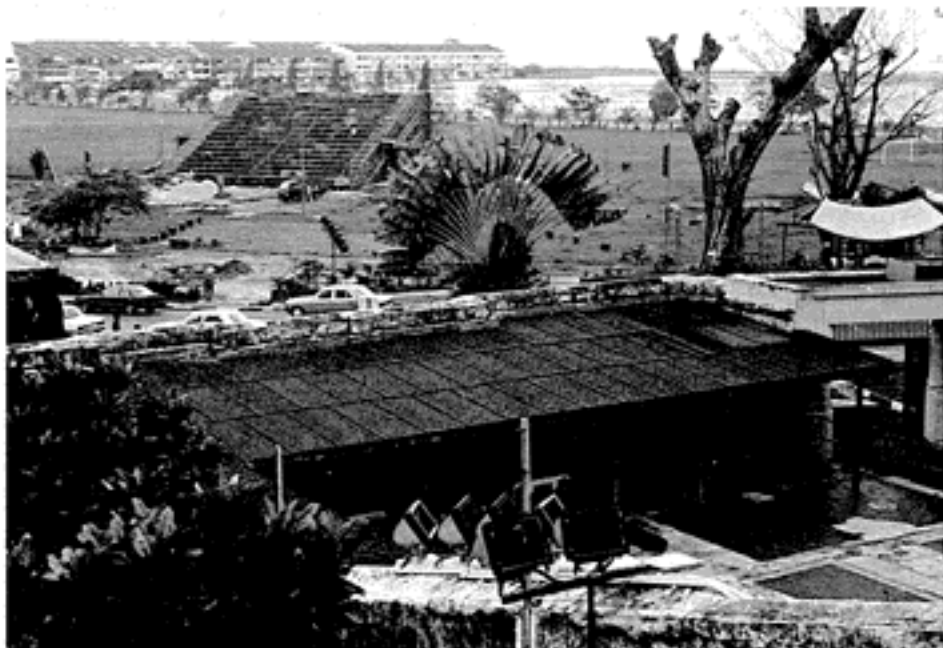
Audience seating stand under construction on reclaimed land. The road in the foreground is closed to traffic during son et lumiere performances.
